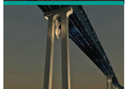
Final designs for the Coronado Bridge lighting project.
